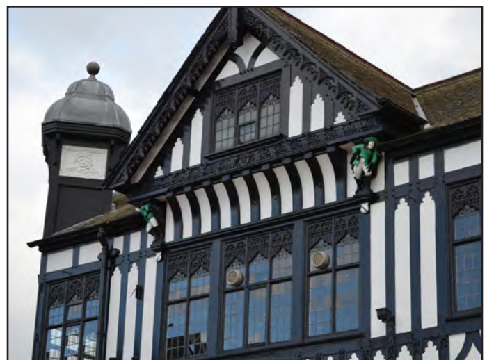
Fig 55: 20-22 High Street. An example of the black and white timber-framed buildings, common in the Town Centre.
