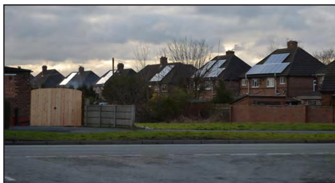
Fig 57: Solar panels on the roofs of Parkfield Road, Witton.
